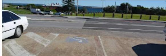
There are more than 50 car parking bays in the area. Two are marked mobility parking bays. The mobility parking area is concrete, 2.6m wide and 6m deep, with a shared 2m gap between the parks.
