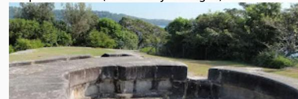
Construction of this initial emplacement took about three years and was completed in 1874. The sandstone pit once had a steel dome (to protect from shells) and was part of a series of gun emplacements protecting from the threat of invasion. Today, you will find a series of tall sandstone channels and the circular pit where the main gun once stood. A set of un-railed steps leads into the pit - please take care in the area, as the pit is not fenced.
