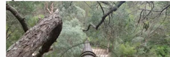
This pipeline is unearthened at Hunter Street, St Ives, and travels through Garigal National Park, across Middle Harbour Creek to John Oxley Drive, Sorlie. The pipe carries water under pressure From Ryde to Pymble to the reservoir at Beacon Hill. The old smaller-capacity pipe can still be seen running parallel to the larger pipe.
