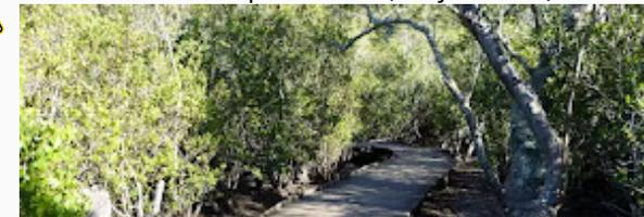
Approximately 120m of elevated timber boardwalk has no handrails, edge capping or markings - there is a risk of falling from the boardwalk. The board walk is 1.7m wide, with approximately 2cm gaps between boards.
