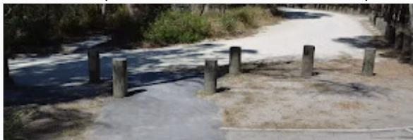
Timber bollard pinch points at the start of the track at the carpark. The gap between the bollards are 1.18m, they are 55cm high.
