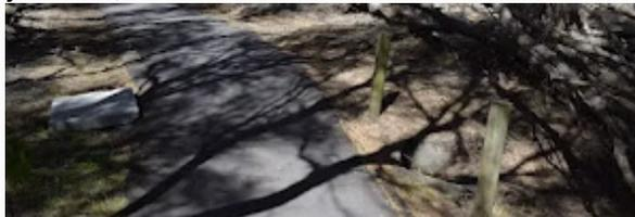
Culvert under path with exposed drainage ditch on the very edge of path. A drop of about 25cm. Marked with timber bollards, there are a series of 4 more similar drainage ditches about every 40m.
